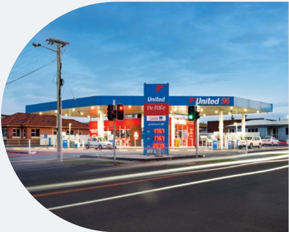
United Petroleum Devonport TAS
