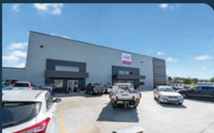
Major Logistics & Food Distribution Centre p. 25
