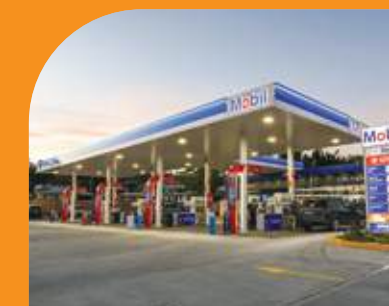
MOBIL FUEL Coffs Harbour NSW
