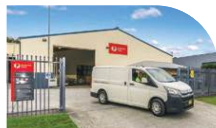
Aust Post Distribution Centre Tweed Heads South NSW
