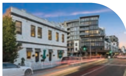
The Exchange Hotel Port Melbourne VIC
